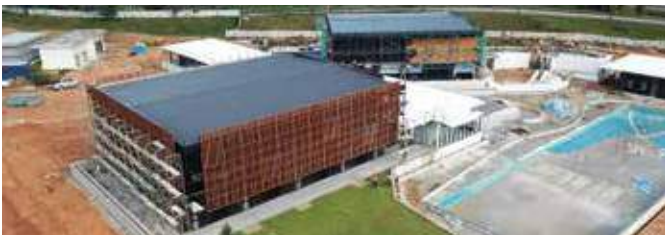
February 2024 Aurora Resort Villas (Clubhouse) Site Progress
