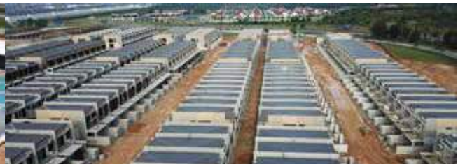
February 2024 Aurora Resort Villas Phase 1 Site Progress
